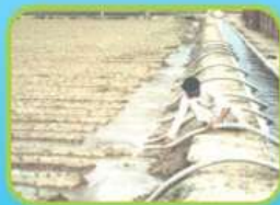
Hydro Flume Irrigation
